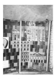
Figure 5.14 Salt damage to the surface of glazed tiles caused by constant leaching of water from above.
