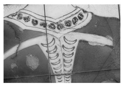
**Figure 3.22** Delamination caused by frost penetration.
