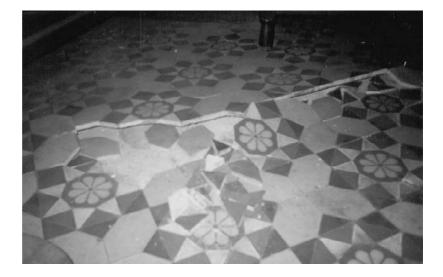
**Figure 5.19** Complete collapse of a tiled floor after severe water penetration.
