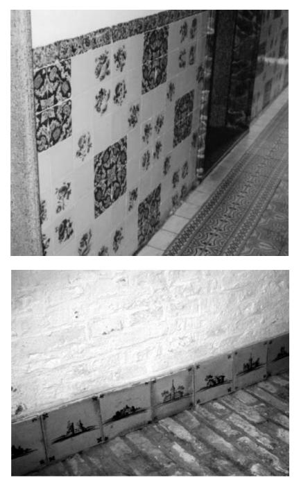
The body clay of delftware tiles was usually dug locally to the site of manufacture; it is rich in calcium carbonate and fine sand deposited as silt from waterways, the addition of marl clay from different locations was sometimes included in a carefully balanced mix which slightly from place to place. Marl is defined as a natural deposit mix of
