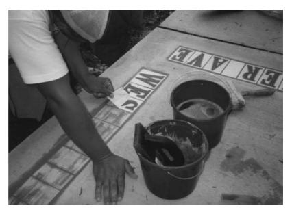
**Figure 7.22** Grouting and removing protective tape from new tiles after installation.
