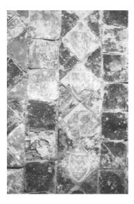
Figure 5.8 Lime encrustations on medieval tiles.
