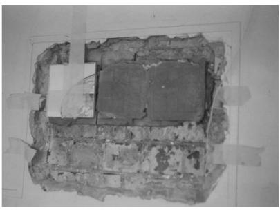
always release the tile, along with its adhesive layer still attached, from the substrate (Figures 5.34–5.36).
