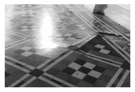
Figure 3.21 Damage caused to tiles under tension by floodwater, the Hallway, Osgoode Hall, Toronto.
