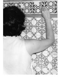
**Figure 7.15** Polyester resin filler being applied to damage.
