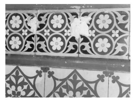
**Figure 7.14** Damage caused by steel pins hammered into tiles.
