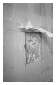
**Figure 3.12** The central tile removed after taping the surrounding tiles safely in position.
