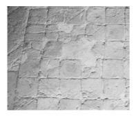
**Figure 5.26** Lime mortar infill in medieval tiles.
