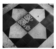
**Figure 2.23** Surface wear to a group of encaustic tiles.
