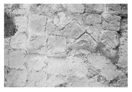
**Figure 3.1** Tiles with footprint in the mortar, the Refectory floor, Denny Abbey, Cambridgeshire.
