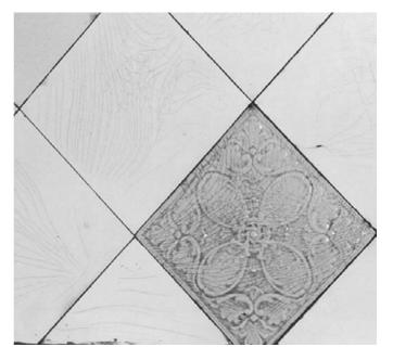
**Figure 5.5** Typical crazing on old glazed tiles.
