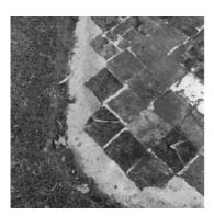
Figure 7.18 Lime mortar 'buffer' zone.
