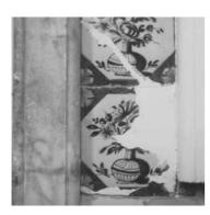
**Figure 5.27** Plaster infill in eighteenth century tiles.
