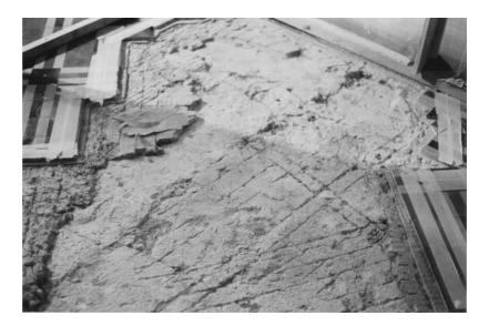
**Figure 7.11** Fracturing in the lower screed.
