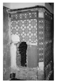
**Figure 7.13** Damage to scheme caused by the letting in of heating ducts to walls.
