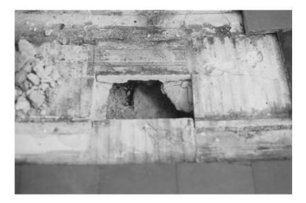
**Figure 5.20** Crumbling lime mortar in a subfloor due to shrinkage of the timber joists.
