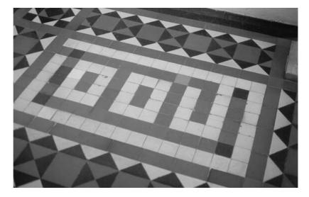
**Figure 7.6** Poor colour matching and inattention to the logic of the design during previous repairs.
