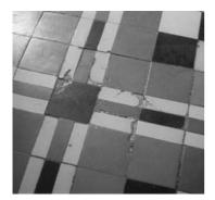
Figure 5.21 Spalled edges of tiles due to tensile pressure.
