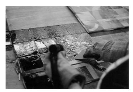
**Figure 7.28** Removing the residue of adhesive with steam.
