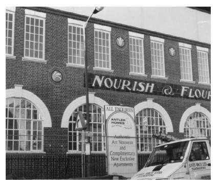
**Figure 5.33** Redevelopment of a baby cereal factory building leaving the original tiled façade in place.
