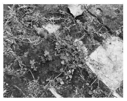
**Figure 7.16** Damage caused by weed growth.
