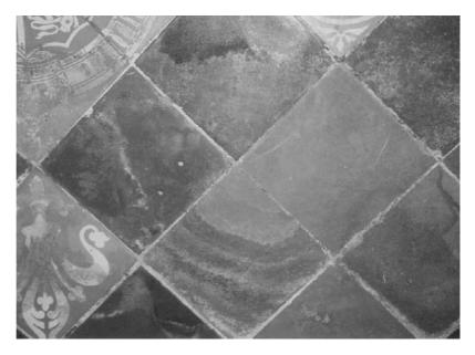
**Figure 5.15** Residue of salt damage caused by slow evaporation.
