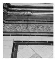
**Figure 5.6** Fracturing caused by building load.
