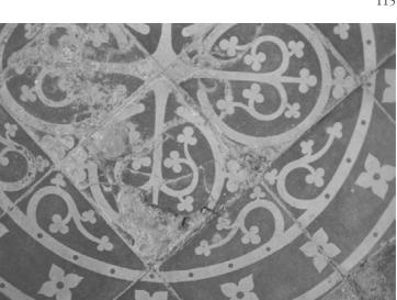
Figure 5.13 Exfoliation caused by salt action on floor tiles caused by moisture leaching from below.
