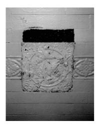
**Figure 5.12** A sample after paint removal.
