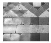
**Figure 5.29** Damage forming a trip hazard in floor tiles at the entrance to a church.
