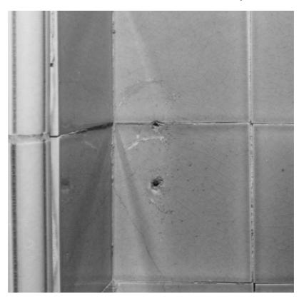
**Figure 5.1** Typical damage caused by drilling into glazed tiles.
