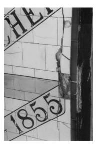
**Figure 5.25** Compressive tension and shifting causing fracturing and misalignment.
