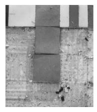
Figure 7.8 Differing sizes found in original tiling which had been cut to fit.
