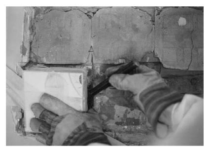
Figure 5.36 Releasing tiles from the substrate with mortar attached.
