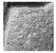
**Figure 7.19** Frost damage on tiles, the result of many years' exposure.
