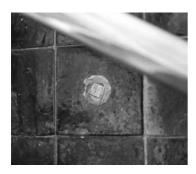
**Figure 5.32** Steel fixings left in glazed tiles.
