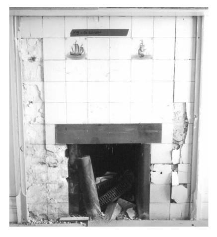
**Figure 5.18** Degraded lime plaster adhesive in a delft tile fireplace.
