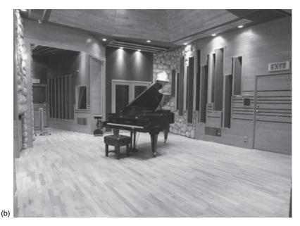
**Figure 7.8** *cont.* (b) Another Toyashima variable room at the Townhouse, London, UK, with semi-cylindrical, rotatable wall panels (Photograph by Bob Stewart)
