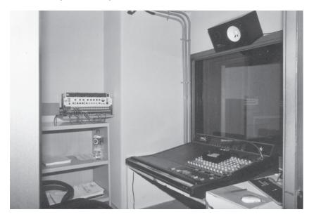
Figure 5.28 An absurdly small 'control booth'. Rooms of such small sizes are effectively too small to allow a flat monitoring acoustic, and colouration is unavoidable
