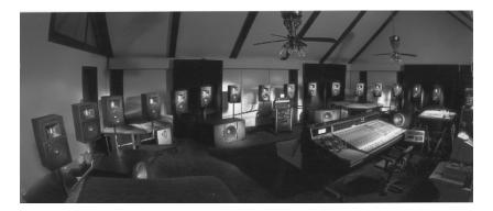
**Figure 19.20** The multi-channel monitoring system in the private studio of Eugene Czerwinski, the founder of Cerwin Vega Inc. The use of one-track-to-one-monitor is said to reduce drastically the levels of intermodulation distortion, and to increase greatly the level of perceived openness and neutralness in the reproduced sound. (Photograph courtesy of Eugene Czerwinski.)
