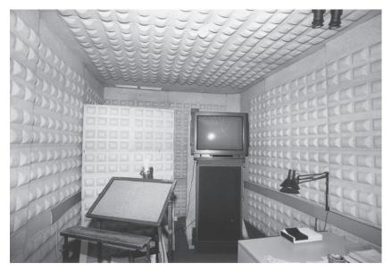
Figure 5.24 A voice recording room constructed without the required space behind the 'absorbent' panels on the walls and ceiling
