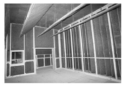
Figure A.1.10 The completed acoustic treatment, viewed from the monitor loudspeaker wall
