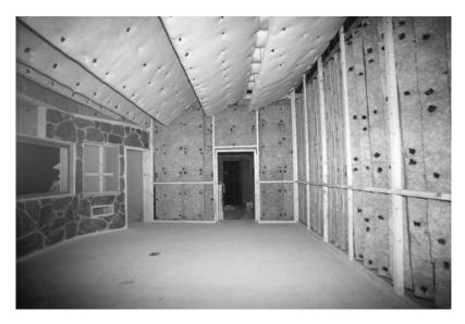
**Figure A.1.11** The completed acoustic control system at Area Master studios, Vigo, Spain; viewed from the rear, and showing the closed nature of the ceiling panels from this viewpoint. Compare this with the view in Figure A.1.12
