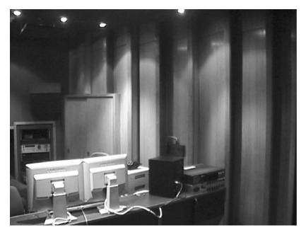
Figure A3.1 View towards the rear of the Jensen designed control room at Sintonia, Madrid, Spain, showing the exposed entrances to the sawtooth absorbers on the side wall
