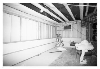
Figure A.1.12 Discosette 3, Lisbon, Portugal; at the stage of mounting the first fabric panels over the absorber systems. The floor is pink marble. The covering on the waveguide panels is Dacron
