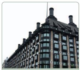
Portcullis House, Westminster, London Architects: Michael Hopkins and Partners, 2001Cooling is assisted by the thermal capacity of the room structures. When external air temperatures exceed 19°C, water from boreholes, at 14°C, is pumped through the air-handling units to cool the supply air down to room temperature (Photo: the author)
