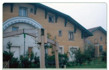
Earth housing at Île d'Abeau, near Lyons, France Construction of a experimental earth housing centre in the 1980s. The project was undertaken by a range of architects including Hugo Houben and has had a major influence on the revival of interest in earth construction (Photo: Howard Liddell)
