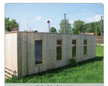
Mader School, Austria A simple plan for a very cheap temporary, selfbuild and movable structure. Walls and roof are made of white pine massive wood construction with orthogonal dowels. The result is very cheap but with nicely detailed finishes (Architect: Walter Unterrainer; photo: the author)
