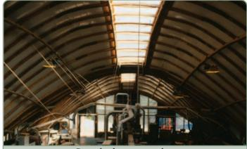
Roundpole construction Much of the early work on roundpole construction was undertaken at Hooke Parke by ABK and Buro Happold (Photo: Howard Liddell)
