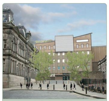
Abertay Life Extension The life of this 1960s University building was proposed as being extended by the addition of an extra floor (Photo Montage: Gaia Architects)
