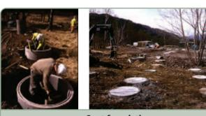
Spot foundations At Glencoe the building was placed on spot or pad foundations rather than a massive concrete slab (Architects: Gaia Architects; photos: Gaia Architects)
