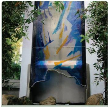
Water wall and planting, providing controlled humidification at Prisma, Nuremburg (Architect: Joachim Eble Architects; Photo: the author)
