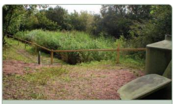
Hybrid System Package plant followed by horizontal-flow reed bed. The reed bed provides buffering and tertiary treatment, reducing BOD and suspended solids to low levels (Photo: Elemental Solutions)
