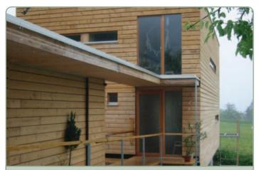
House at Batchuns, Austria One of an increasing number of houses built to a passive standard from Brettstapel construction (Architect: Unterrainer, Photo: the author)
